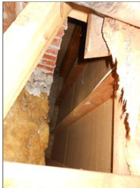
4.1 Picture 3 Area around chimney
