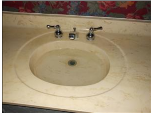
6.1 Picture 2 Master bathroom sink holds water
