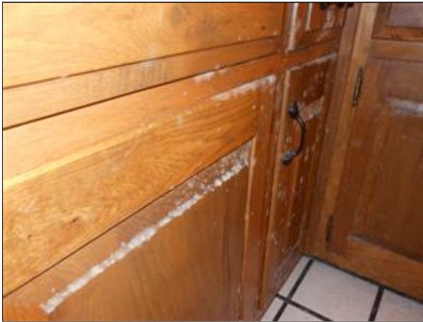
4.3 Picture 1 Mold on cabinets
