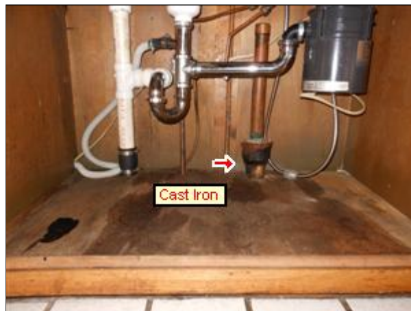
6.0 Picture 1 Cast iron drain pipe
